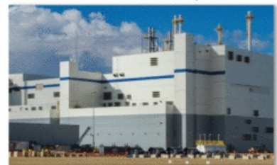
Customer Processing Plant
